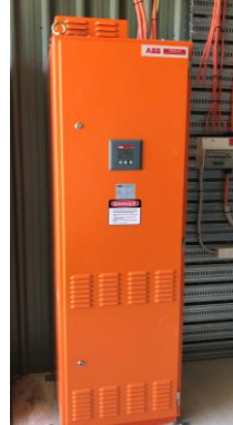
Together with a 200 kVar ABB Power Factor Correction unit.
