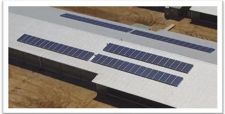
East West Solar Configuration 200kW Solar
