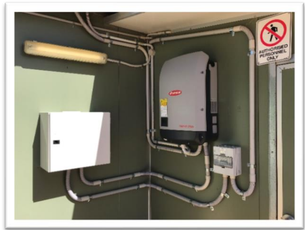
Fronius 20 kW Inverters x 8
